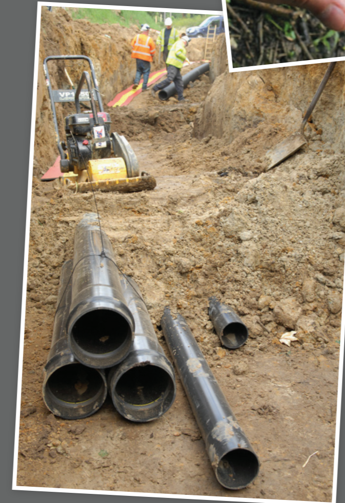
At 22.6 kilometres, the cable transporting the power from landfall at Weybourne beach to the new substation is the UK's longest underground high voltage cable. It was installed using both open trenching and horizontal directional drilling.
