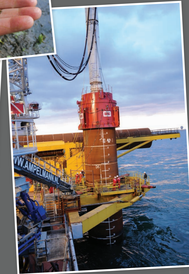
Foundation installation began in June 2010 and was completed just over a year later in August 2011. Each foundation was made to individual specifications and weighed from 375 to 530 tonnes.
