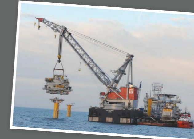
The state-of-the-art crane vessel Oleg Strashnov installs one of the two 900 tonne offshore substations – a key milestone for the project.
